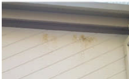
Figure 3. Carpenter bee staining on hole in fascia.
