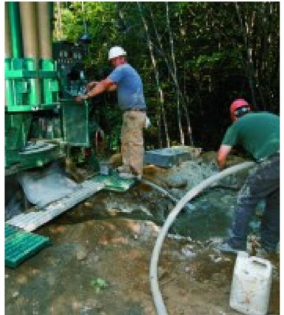
This photo shows a mud pit. A non-porous bentonite clay and water mixture is poured into the hole as it is being drilled. This forces the drilling fines out of the hole. Think of the wood chips that come out of holes drilled in wood, only the size of these “earth chips” and the depth of the drilled hole make the mud necessary to clear the debris.
